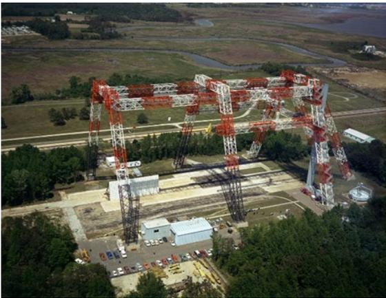
**Figure 5. (Left)The Lunar landing research facility with the cranes supporting the lander can be modified to execute ground test for the testbed.**
