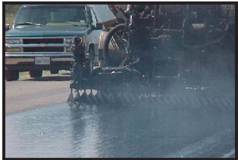
Figure 2. An Asphalt Distributor at Work
