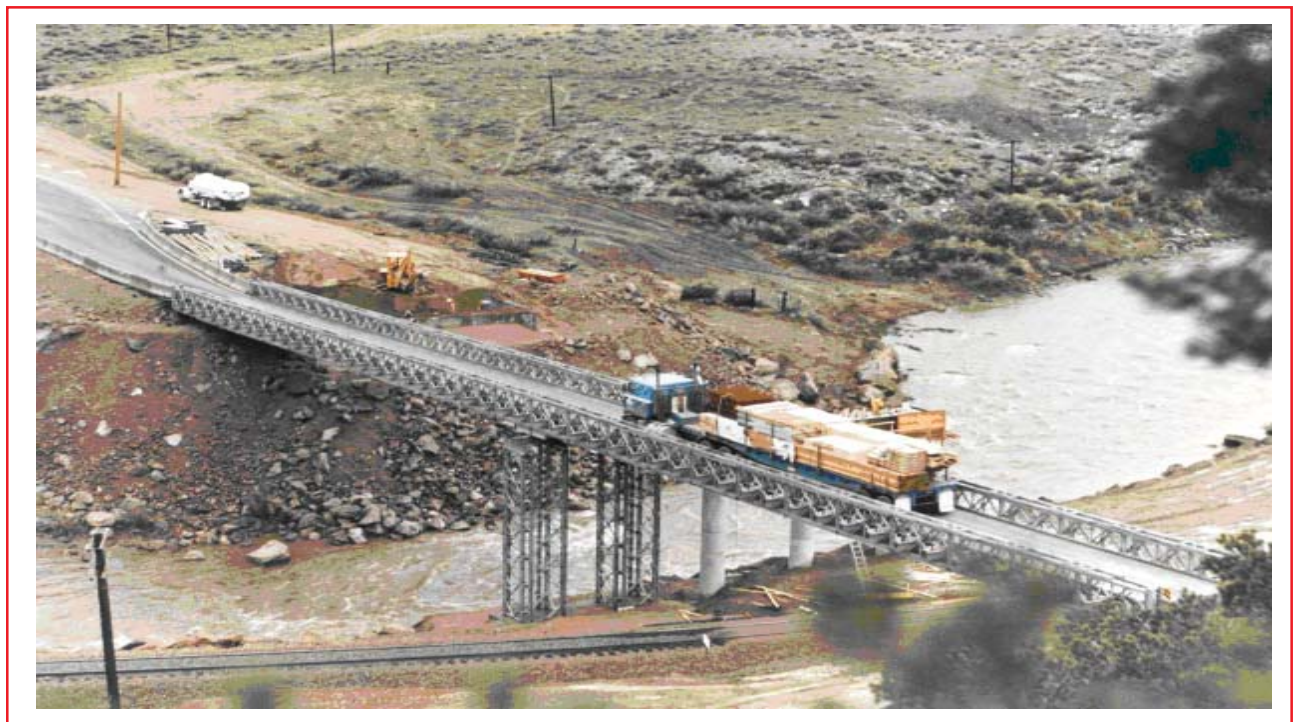
Figure 2. Acrow Temporary Truss Panel Bridge and Supports (Provided by Acrow Corp.)
