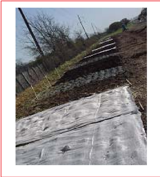
Figure 2. Example of the Falls County test site immediately following installation.
