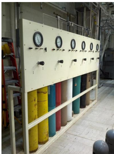
Figure 2. Gas Supply Assembly for S-Bosch.
