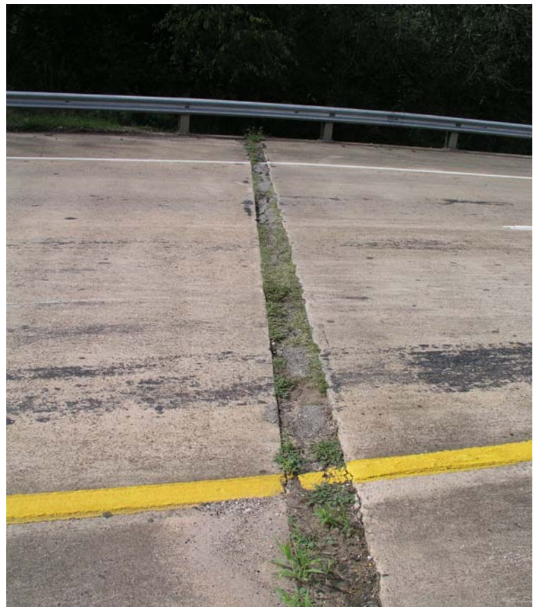
Figure 2. Poorly Maintained 5-inch Wide Joint Between Bridge Deck and Approach Slab.
